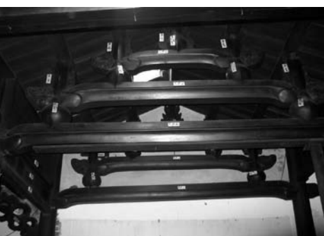
“Chong ruong” rafter, a wooden structural component of traditional houses in Hoi An (Photo: HACMMP)
