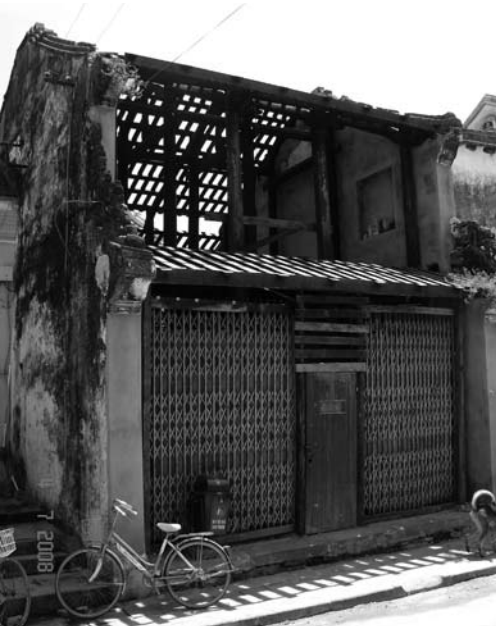
Inappropriate materials, such as iron grill doors are being used in the partial restoration of some old houses (Photo: HACMMP)
