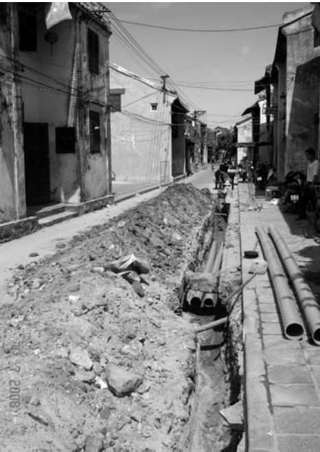
Sewage pipes are just starting to be installed within the historic core zone (Photo: HACMMP)
