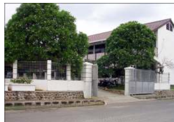
UPT Administration office
